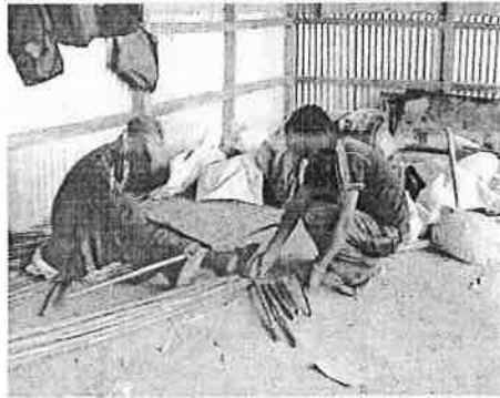
Fig. 4: Bamboo spacers used for perimeter holes
