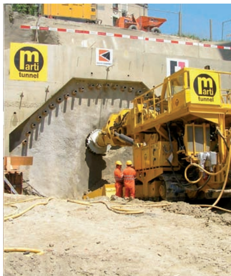
Road header excavation
