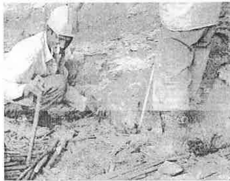
Fig. 5: Charging of blastholes with bamboo spacers
