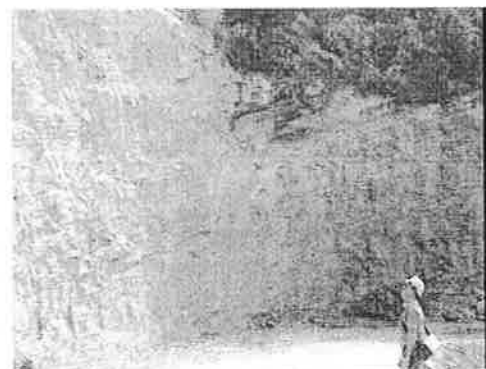
Fig. 9: Final wall obtained through controlled blasting using bamboo spacers
