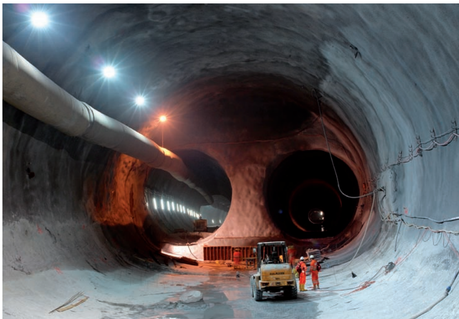
Twin tube tunnel
