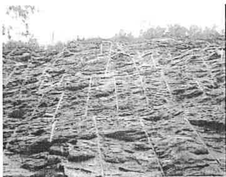
Fig. 8: Half-cast factors obtained with bamboo spacers
