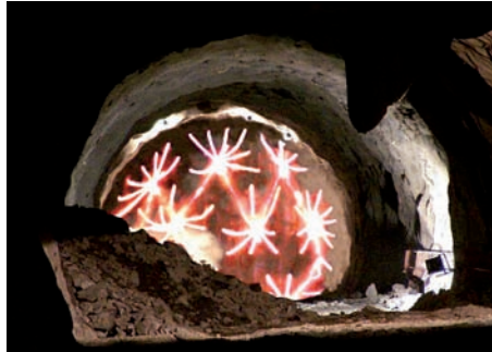
Drilling and blasting, full face
