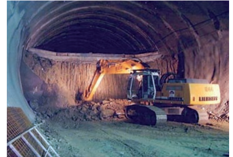
Mechanical excavation, top heading bench
