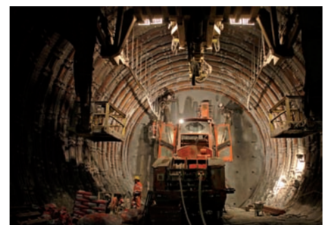
Conventional tunnelling in squeezing ground (full face)
