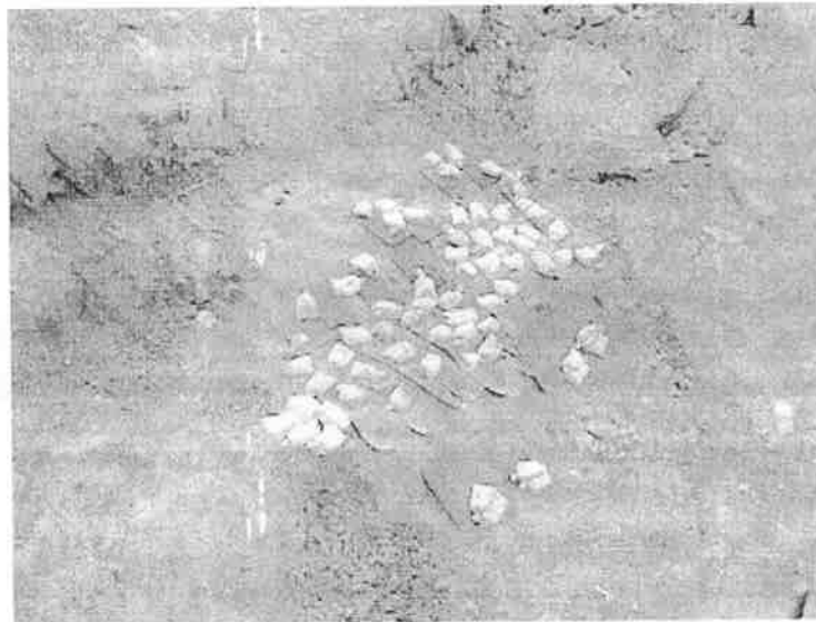
Fig.6: Muffling arrangement with conveyor belts and sand back at Millennium Centre, Aizawl Town, Mizoram
