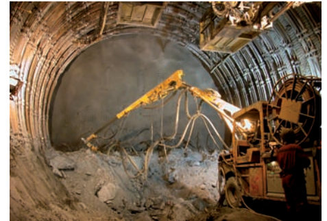
Face support with shotcrete
