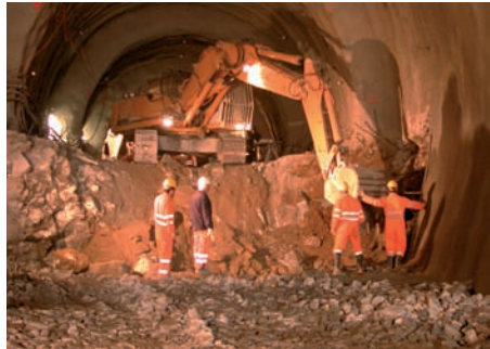
Excavation with shovel
