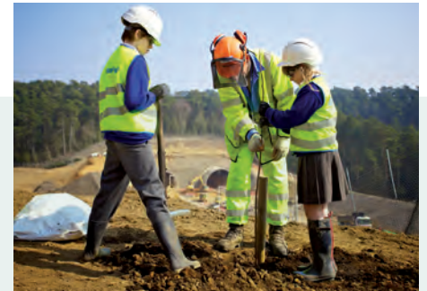
Figure 21 : Stakeholder management with the youngest in UK ® A3 Hindhead Tunnel
