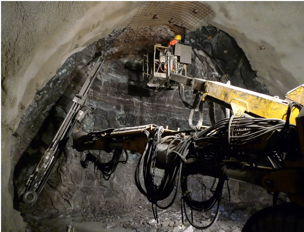
Fig. 2: Pilottunnel in hard rock conditions
