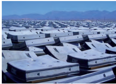
Figure 8 : Stored precast concrete segments ready for supply to the tunnelling work for a water supply project. The logistics and supply of this type of tunnel support are extensive and needs to be considered early in the tunnel planning phases. © Daetwyler
