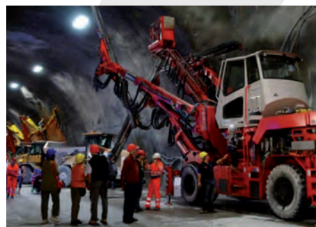
Figure 16 : Open site event attract all generations (© AlpTransit Gotthard Ltd.)
