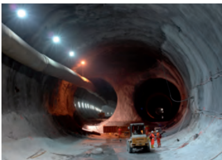
Figure 4 : - Top: Drilling jumbo working in a conventional tunnel drive. - Below: Tunnel bifurcation excavated by conventional tunnelling General description of the project development process © AlpTransit Gotthard Ltd.
