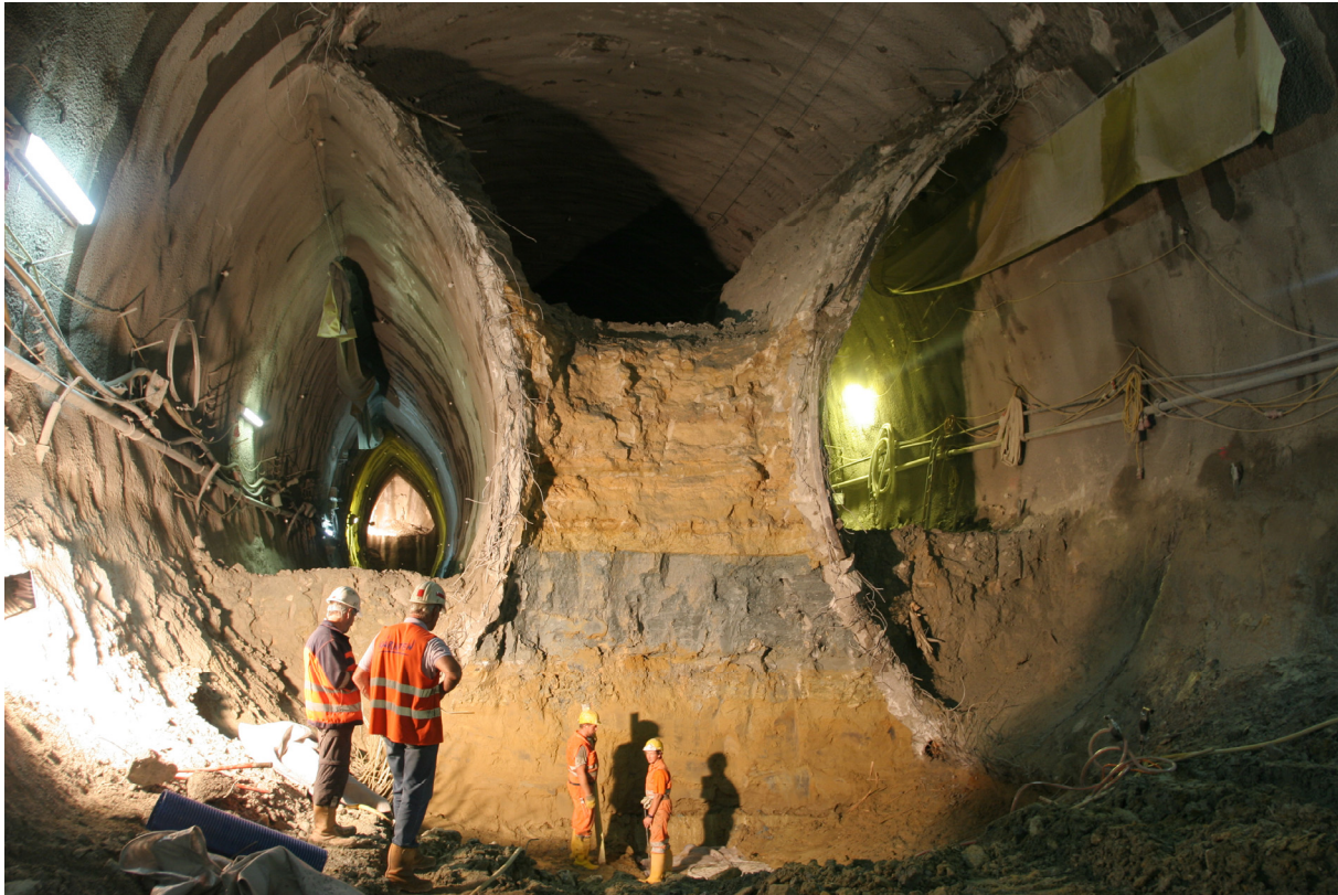
Fig. 12: Double-track railway tunnel in urban environment
