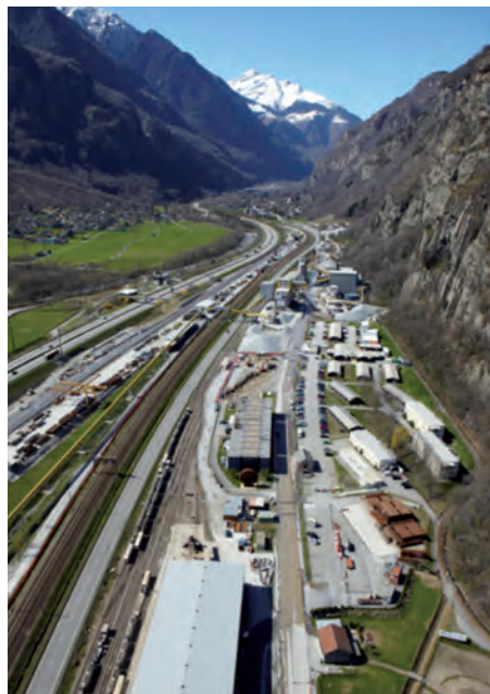
Figure 18 : Rig area of a major tunnel project - the heart of logistics® ATG
