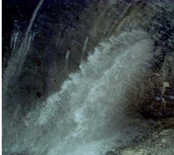
Figure-2: Early warning information for critical ground while TBM boring reduces hazardous geo risks like enhanced water-inflow
