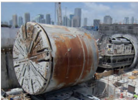
Figure 2 : Top left: Lowering a TBM into the start shaft Lower left: TBM arrived at the portal with back-up still inside the tunnel © Babendererde Eng
