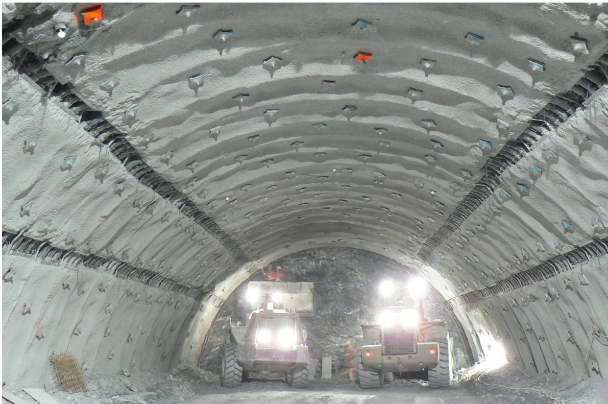
Fig. 4: Yielding elements installed in longitudinal slots in the top heading
