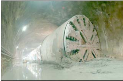
(A) Partial invert excavation
