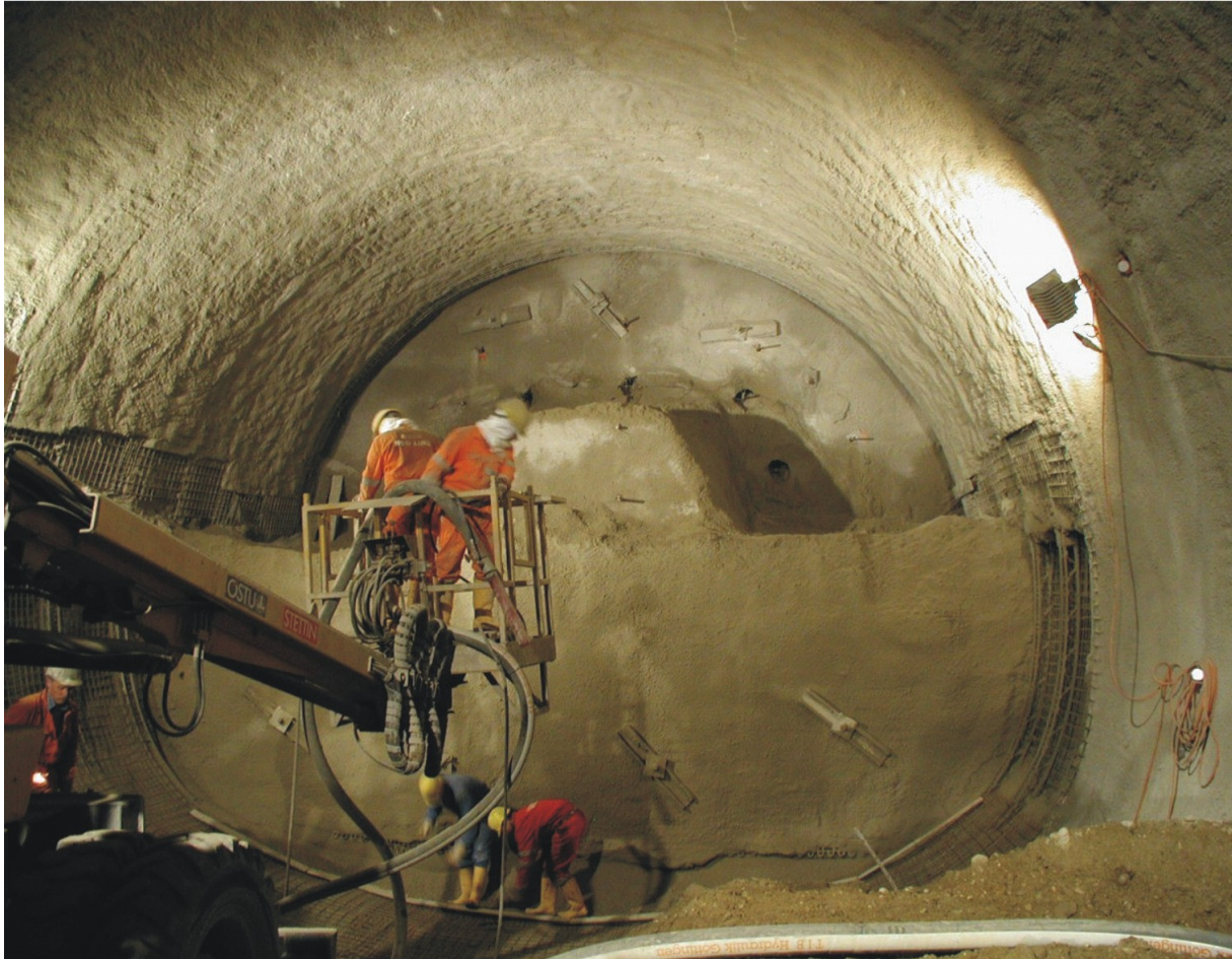
Fig. 10: Metro tunnel in soft ground conditions
