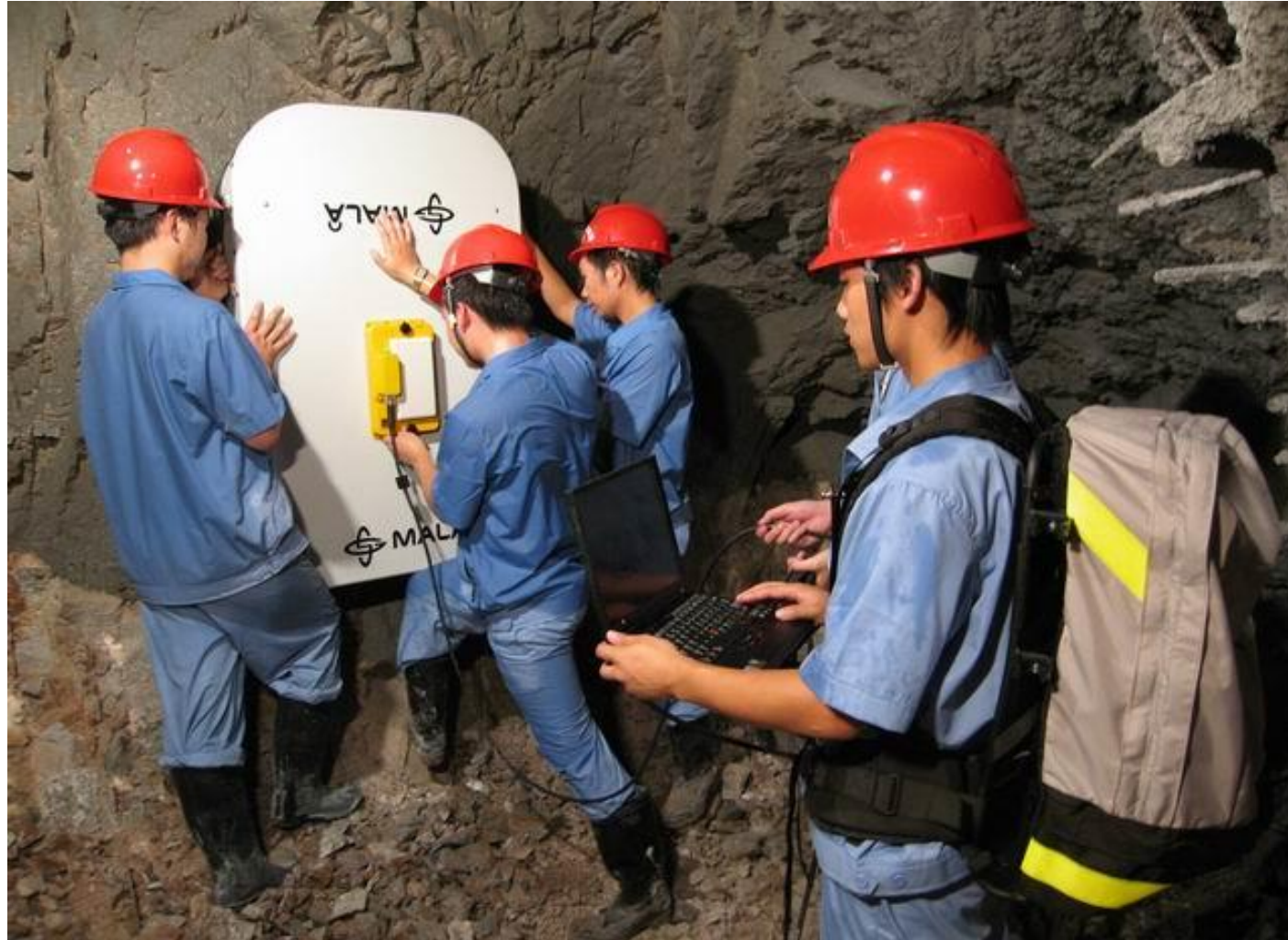
Tunnel forehead using 100MHz shielded antenna Now we can use GX80 or GX160
