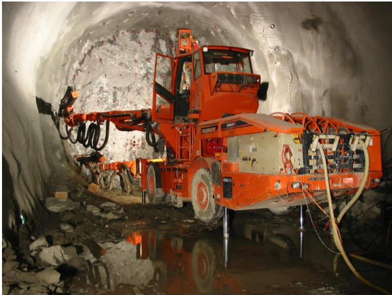
D&B excavation, jumbo perforation and anchor drilling
