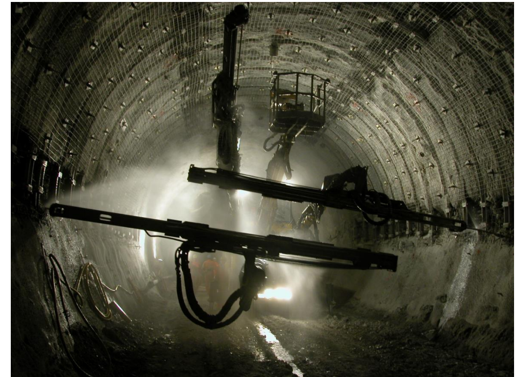
D&B excavation, jumbo perforation and anchor drilling
