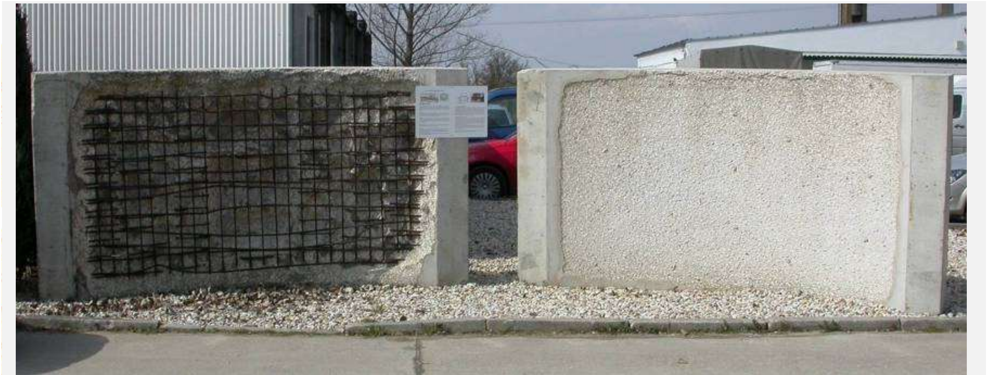
Plain Concrete 340 Mm Spalling Depth (RABT Fire Curve)
