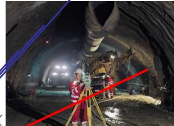
3-D deformation monitoring
