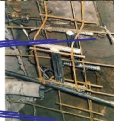
Shotcrete strain meter Pressure cells
