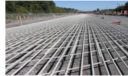
Continuously reinforced concrete pavements (CRCP) in Roads
