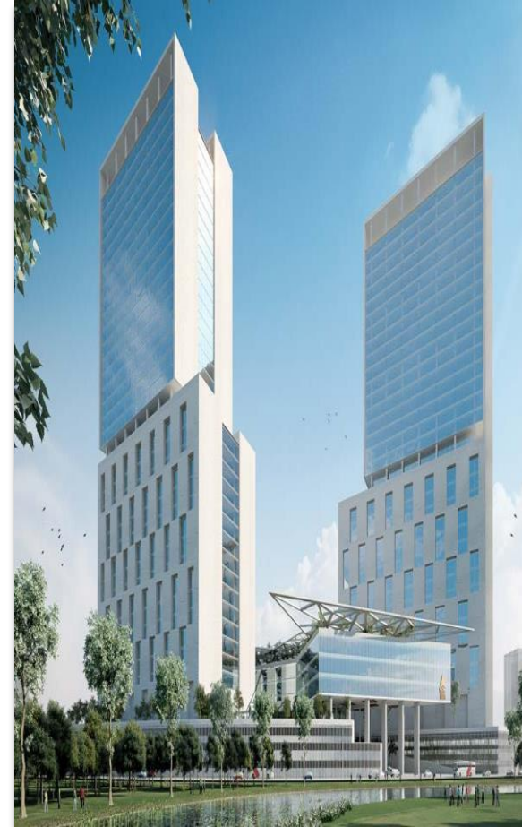
Sands Infra – IT Office Tower Kochi SmartCity
