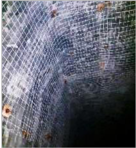
Welded wire mesh with rock bolt used on mine roof
