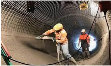
Shotcrete works done for protection of linings in Tunnels
