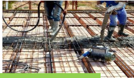
Screed flooring for slabs made of Precast girders in Metro Projects
