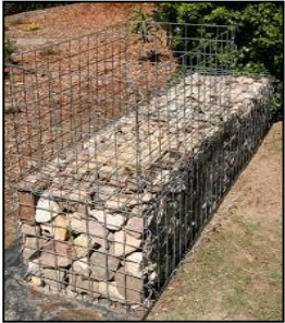
Gabions – Stone walls
