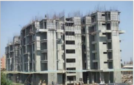
Modern formwork –Walls
