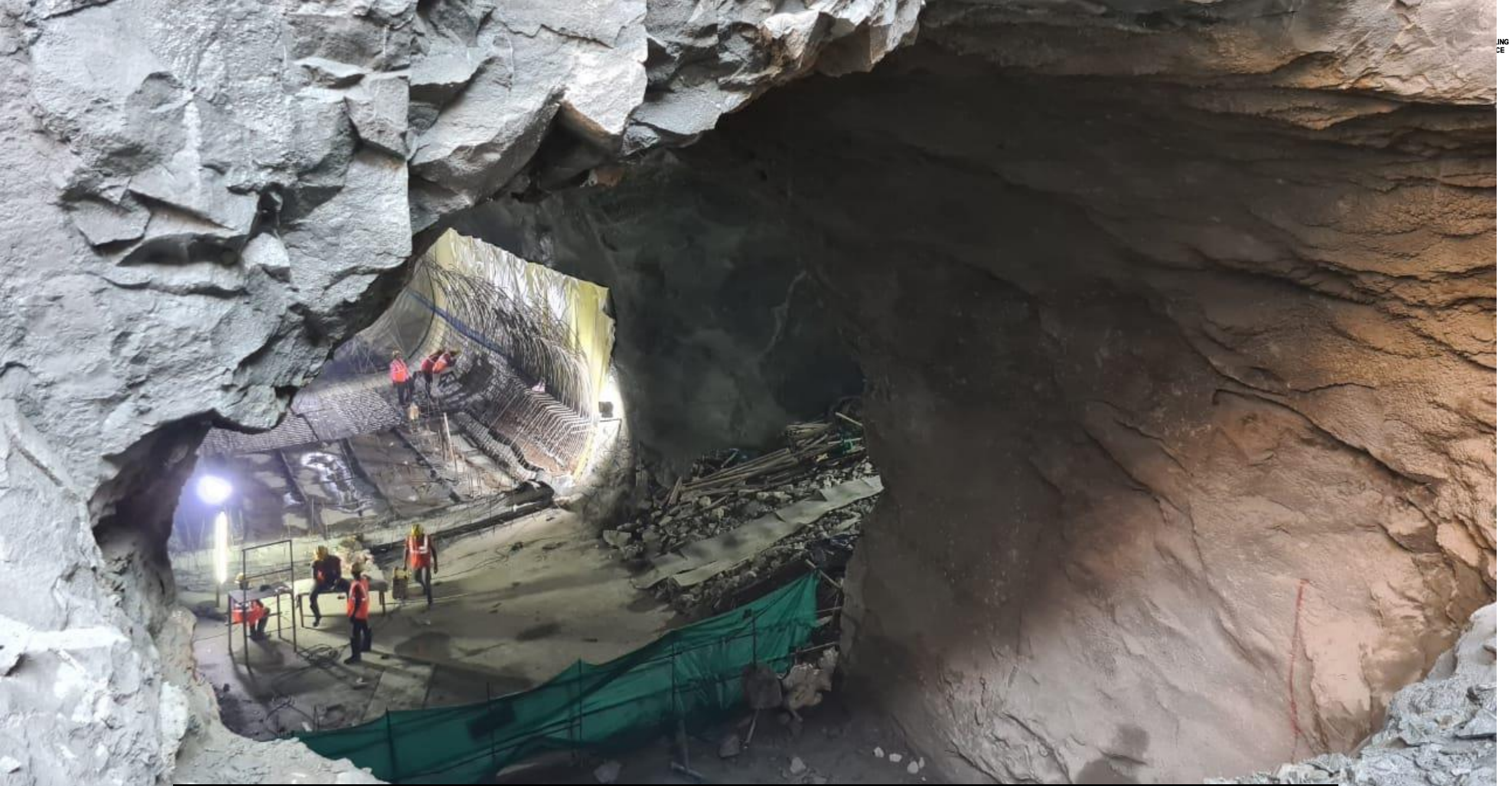
KALBADEVI METRO STATION – OPENING TO CENTRAL CAVERN FROM K2 BLOCK
