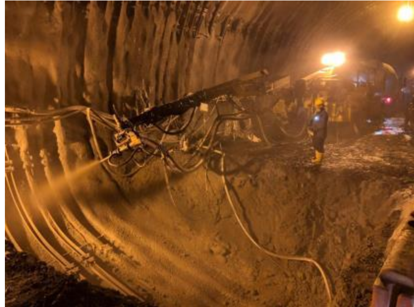
Shotcrete and invert Steel Sets K4+683 a K4+685
