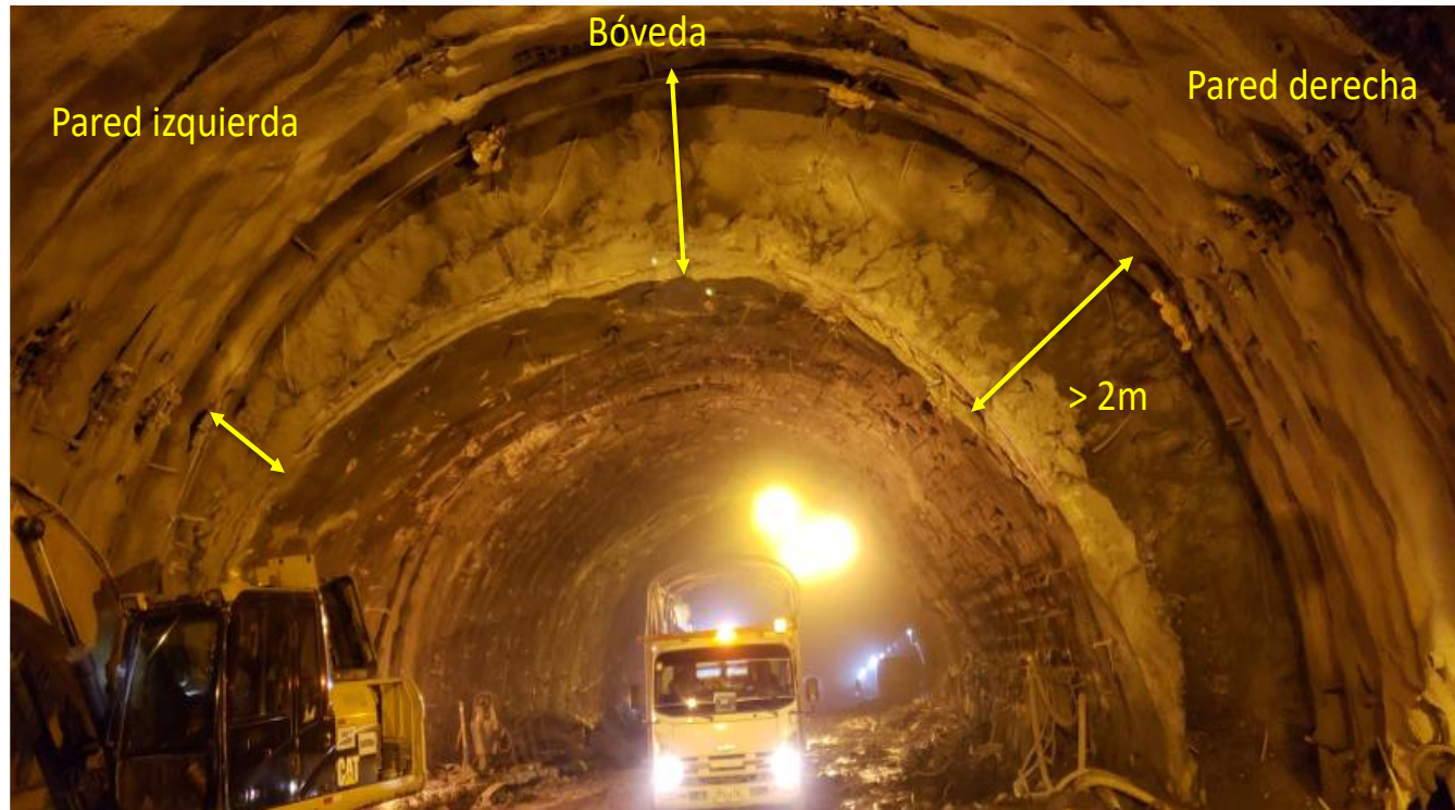
Measured convergence in the main tunnel
