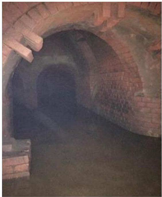
Photographs of existing brick sewer drains
