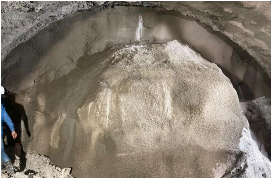
Face Butt at T01 P1 Tunnel Face
