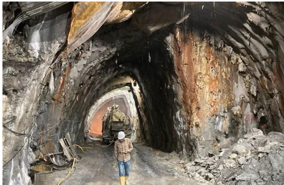
T01 P2 Tunnel Face
