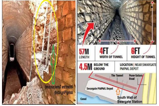
A buried tunnel punctured at the south head wall during the piling activity at swargate station.
