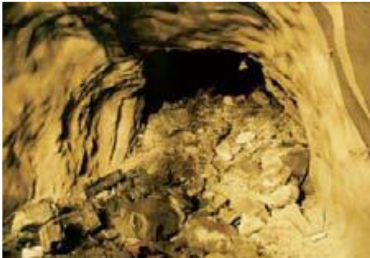
(a) Rock Fall in Laedral Tunnel; (b) Support protection using rock bolts, SFRS and RRS
