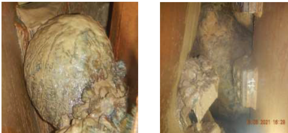
Fig. (4) Boulders from excavation face
