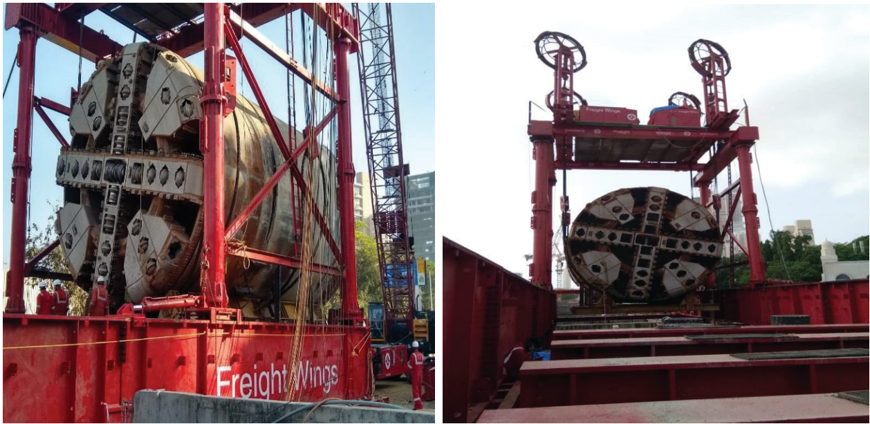
Figure 7: TBM lowering operations using Strand Jack Gantry system at UGC03
