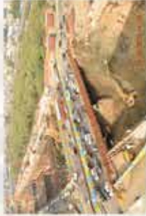
Extensive use of temporary traffic deckings
