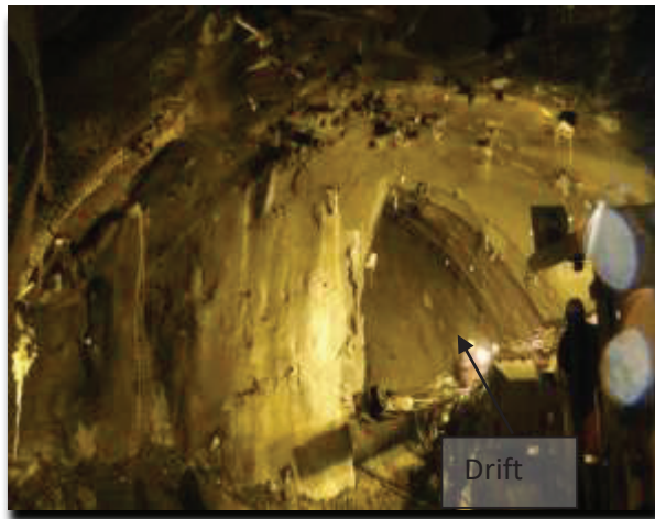
Fig 8: Drift method of tunneling in loose strata at ch 2410.
