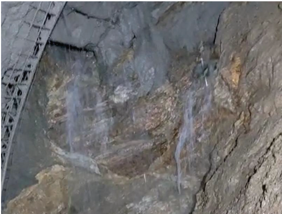
Face Collapse due to heavy ingress of water
