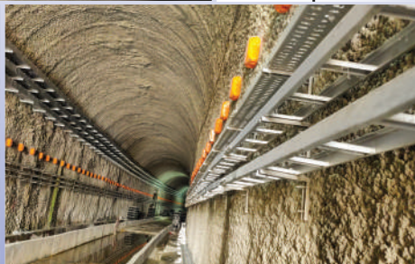
Cable Trays Usbri Railways Tunnel Project, J&K
