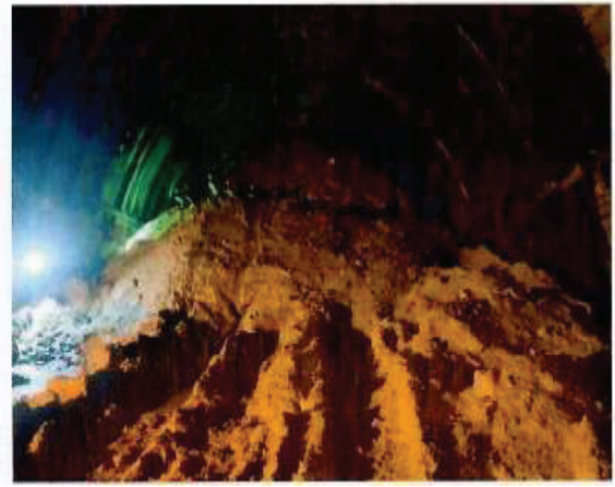
Figure 6: Deposition of muck in front of face-7
