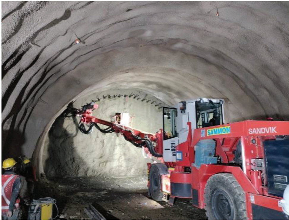
Figure 6: Pipe Roofing in Progress
