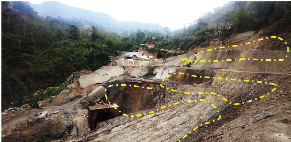
[Fig. 2: Stability problems on slope of Portal 1 of Tunnel T-10]
