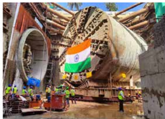
(b) 180 degree skidding work on TBM
