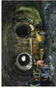
Use of Steel Fibre Reinforced Spayed Concrete (SFRC) permanent lining for a NATM cavern - an innovative first for any railway tunnel in the country
