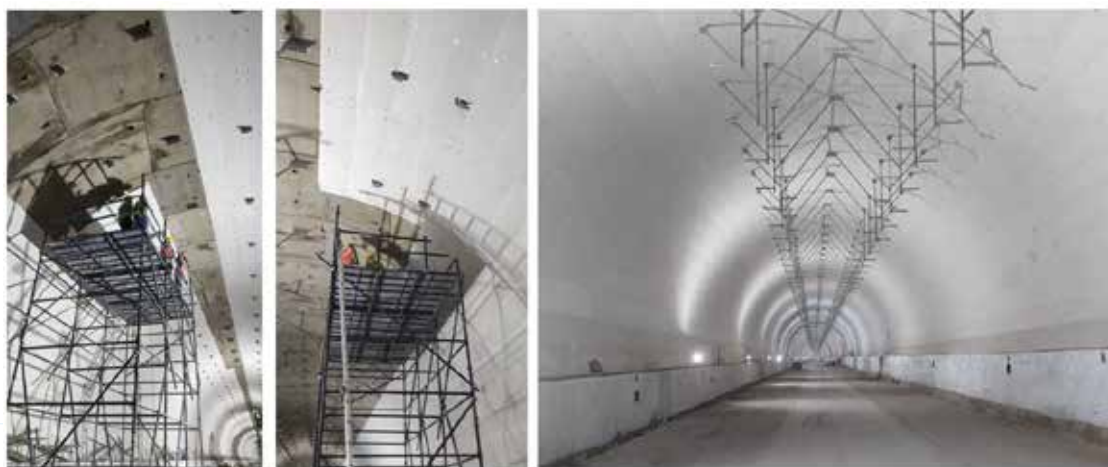
(a) Fire board installation
