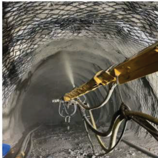
Figure 8. First 20mm shotcrete applied over Dolenco Drain in cross passage
