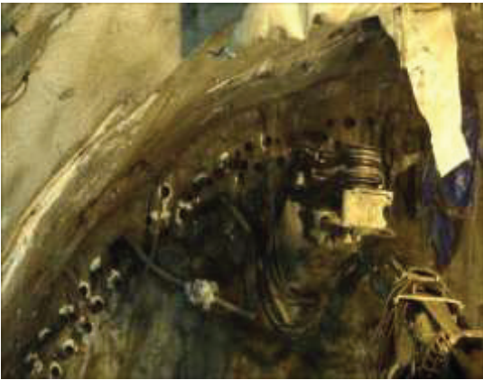
Fig 6: Pipe roofing umbrella (Double layer)
