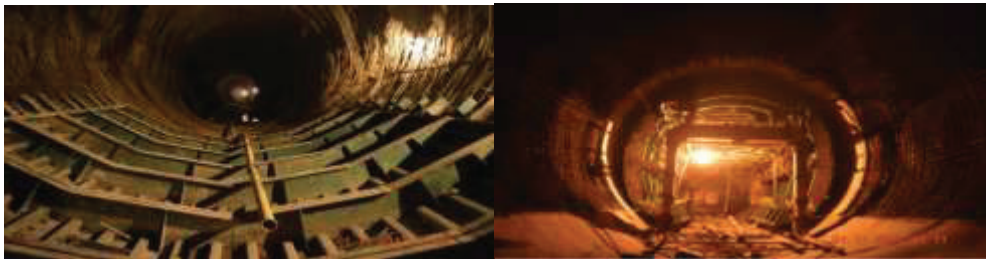
Figure 8. Invert and Overt Rebar and Gantry Shutters
