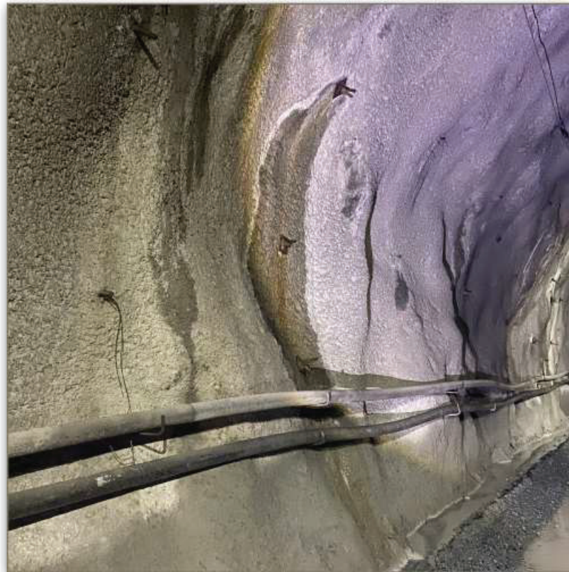
Figure 3. Initial shotcrete layer applied onto the rock surface
