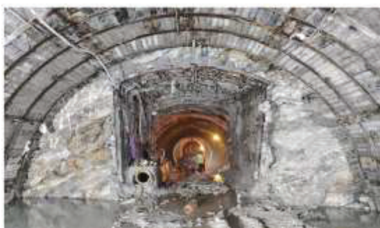
Figure 10 : Widening of central Gullet with Safety Pipe at left side.
