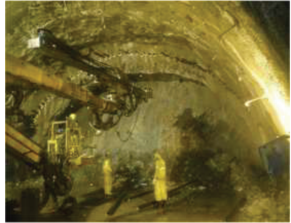
Fig 5: Pipe roofing umbrella (Single layer)
