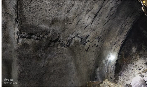
Overstressing of Shotcrete and distortion in LG
