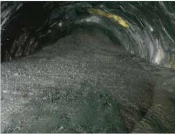
Fig 4: Flow of face at Ch 2077
